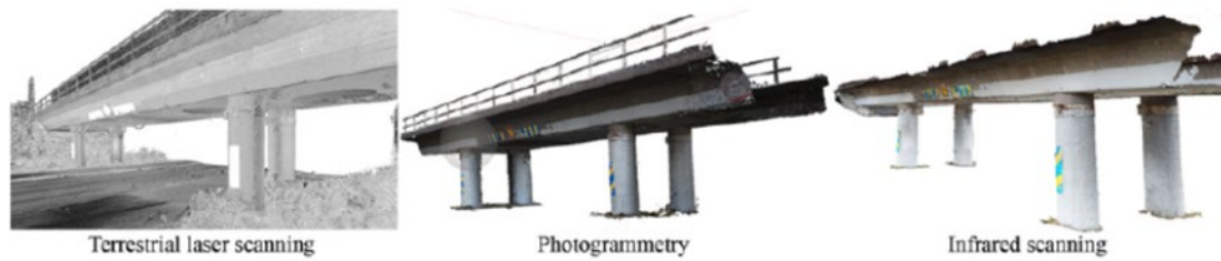
Figure 8: 3D Models of Kalkallevagen bridge – showing different levels of detail obtained between TLS, CRP and IS (from Poposecu et al. (2019))
