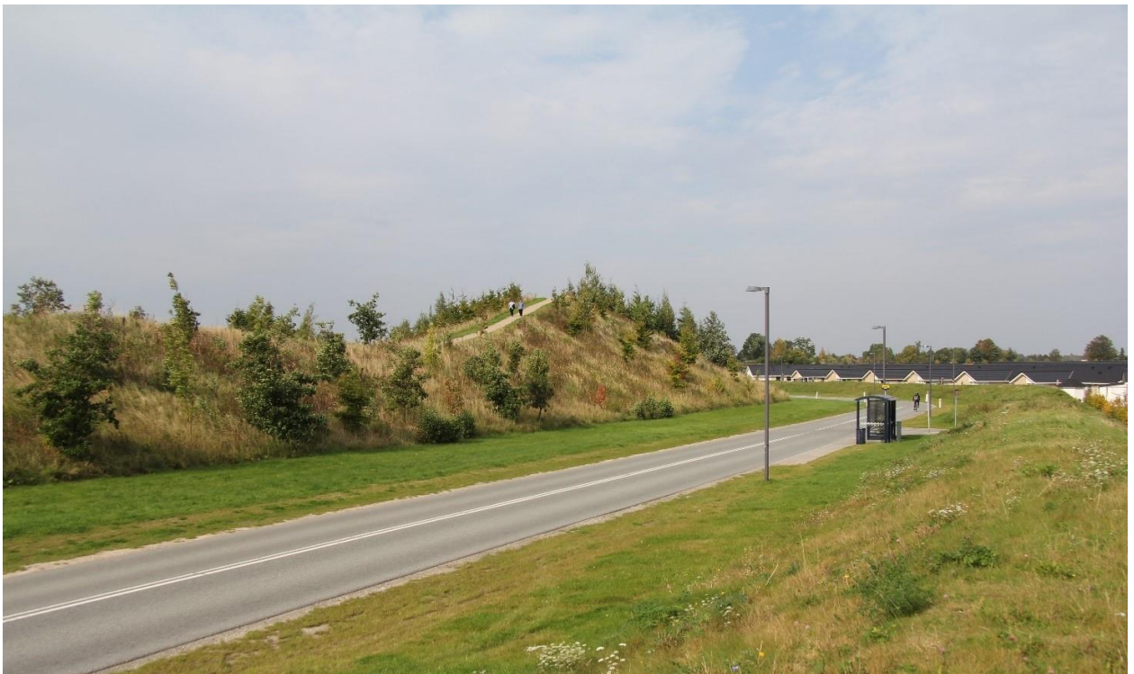
Figure 132: Embankment covering the view to a motorway (not visible on the left), also improved with greenery.
