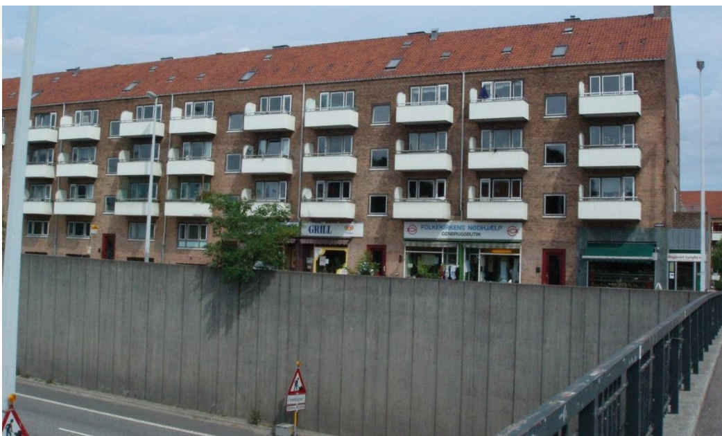
Figure 136: One facade facing the noise from the 6-lane motorway in the front, with chance to a quiet side on the far side. Typical two-room apartments, balconies suggesting living rooms on the loud side, giving a quiet side for bedrooms.
