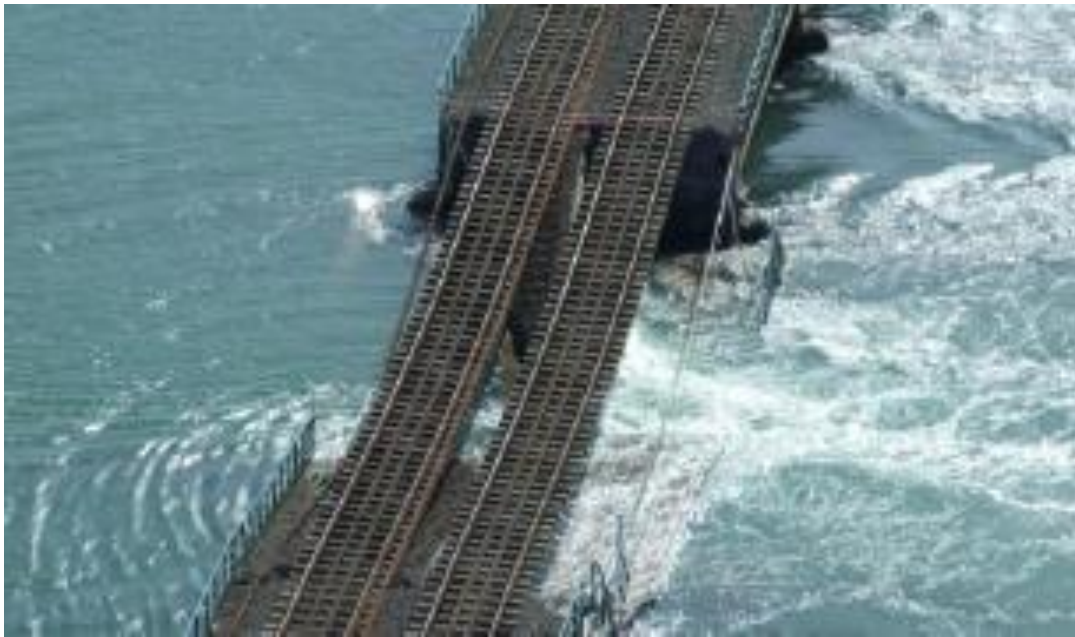
Figure 15 Collapse of Broadmeadow Estuary Bridge Dublin August 2009 (image courtesy Irish Rail)
