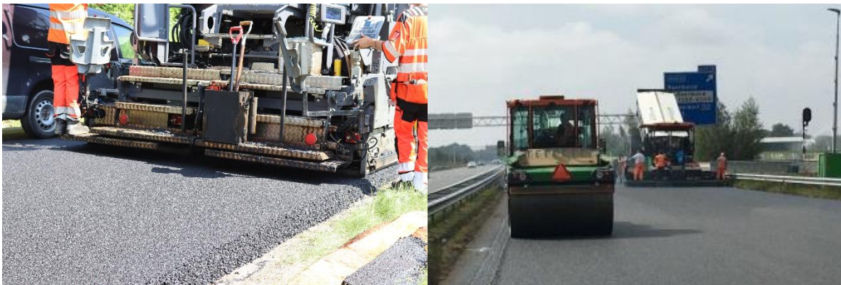
Figure 8. Laying and compaction of FIBRA mixtures
