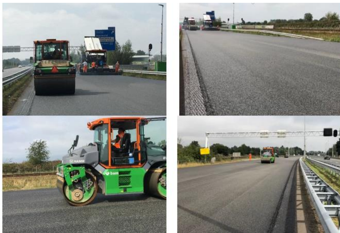
Figure 20. Laying and compaction process of FIBRA mixtures
