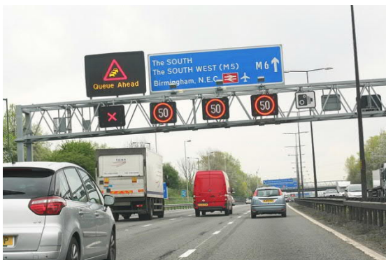
Photo 4.3: Highways England Smart Motorways Gantry, Lane Closure Signs and Signals
