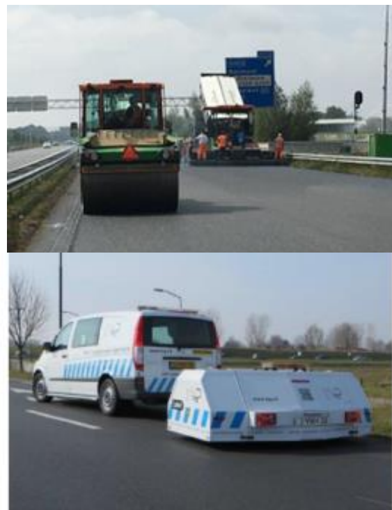
Figure 19. Laying and compaction of FIBRA mixtures (Top). CPX Noise measurement (Down)
