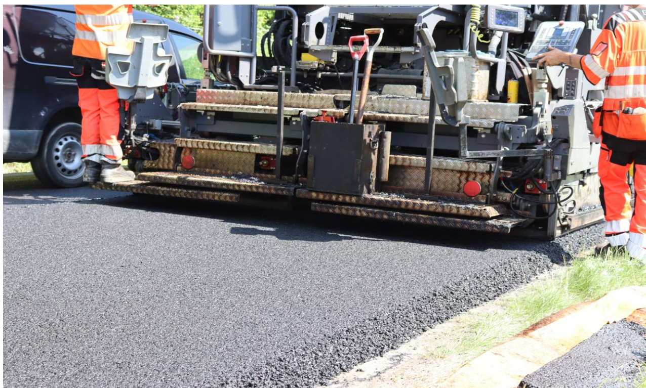
Figure 2. Pilot section implementation (Norway)
