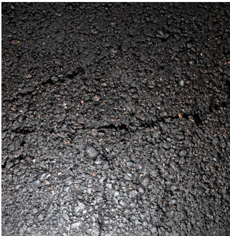
Figure 5-5 Cracks after 120 000 laps in SMA 8 60 % RA, long term aged.
