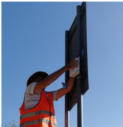
Figure 21. Sensors installation (phases F to J): a) sensors installed, b) sensors and cables, c) sensor covered by cold recycled mortar, d) cables blocked with cementitious mortar, e) data logger installation, f) sensors connected to the data logger.
