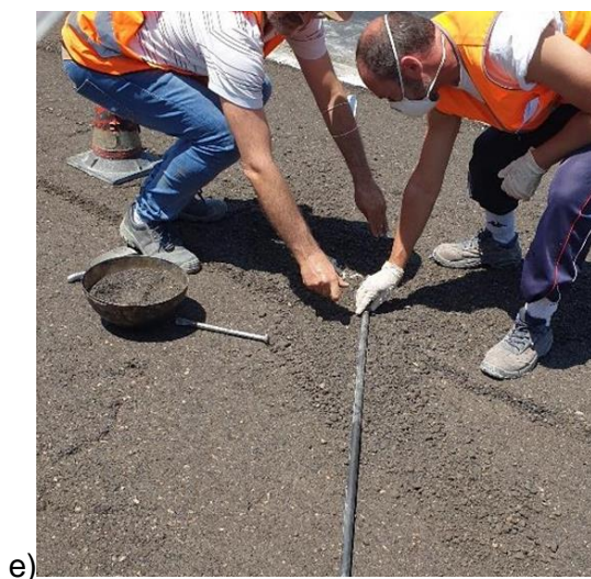
Figure 20. Sensors installation (phases A to D): a) wooden tablets before installation, b) cables covered with flexible metallic tubes before installation, c) positioning of the steel bars d) to f) positioning of the tablets
