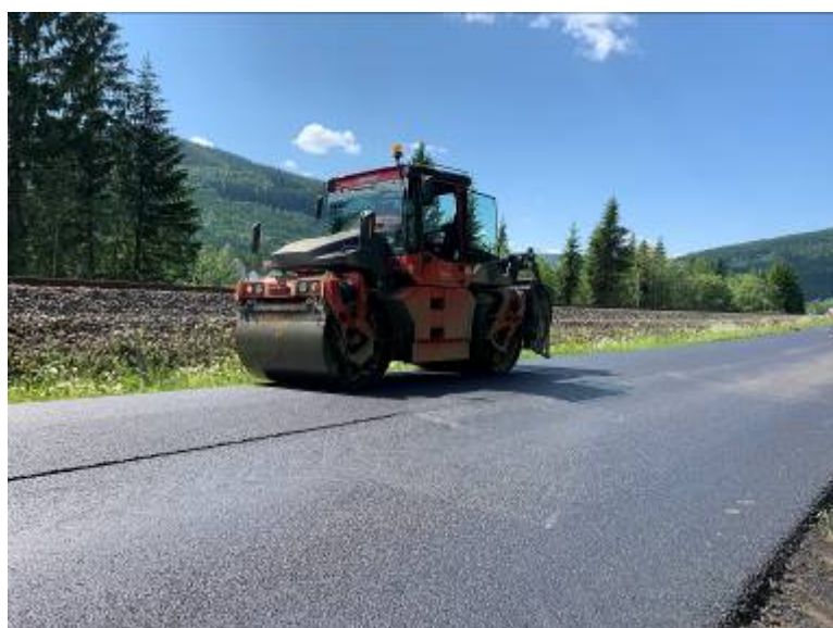
Figure 14. Illustration of compaction process of FIBRA mixtures.
