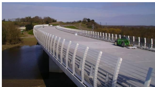
Figure 41: Sound reflecting NB curved to reduce the negative effect of sound reflections
