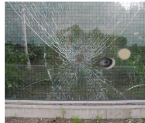
Figure 6: Net-like crack with a hole in a transparent barrier ©BAST, Germany
