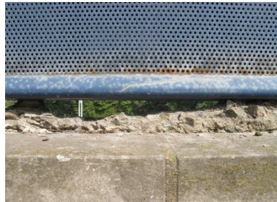
Figure 2: Slit-like leak between an aluminium noise barrier and foundation ©Walloon Road Administration, Belgium
