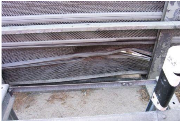
Figure 1: Damage at an aluminium noise barrier after traffic collision ©BMVI, Germany
