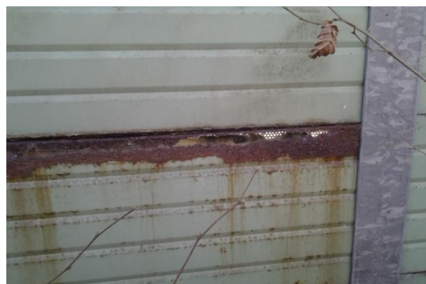
Figure 5: Slit-like leak in an aluminium noise barrier due to corrosion ©Walloon Road Administration, Belgium
