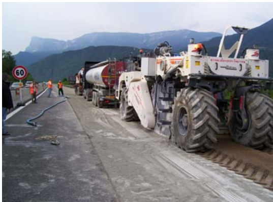
Stabilization with bitumen emulsion
