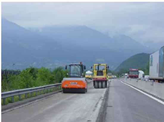
Compaction by means of steel and pneumatic tire rollers
