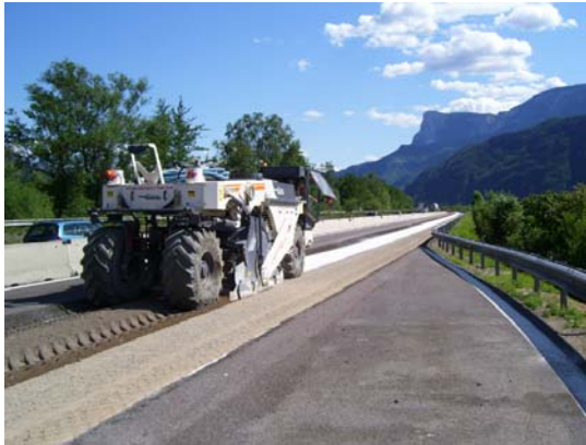
First recycler pass for mixing Reclaimed Asphalt (33%) with the underlying reclaimed aggregate (67%)
