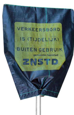
Figure 18. Covering restrictions when work shift is over.
