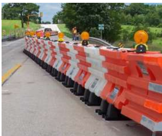
Figure 23. Water-filled portable vehicle restraint systems. Source: www.jtitraffic.com
