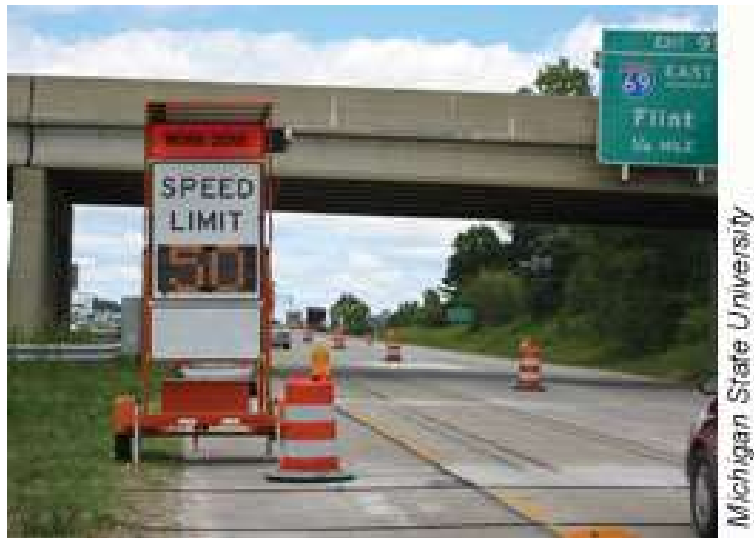
Figure 24: Variable speed limit sign in work zone
