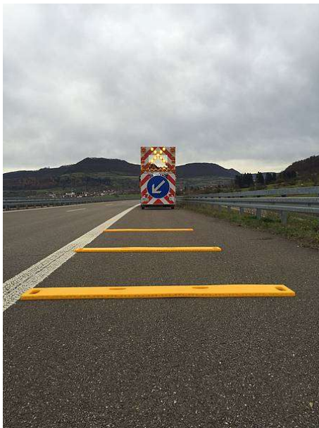
Figure 19: Portable rumble strips on hard shoulder
