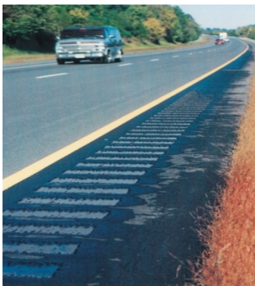
Figure 5.2: Example of rumble strips
