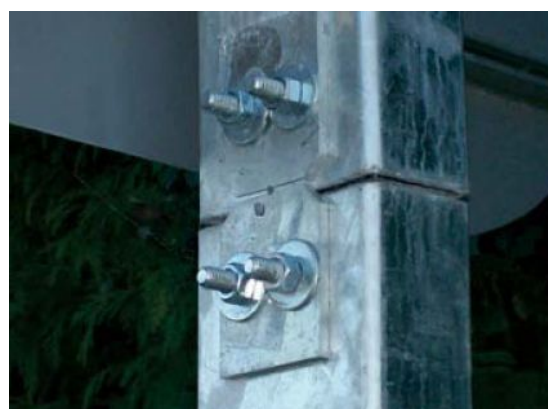
Figure 5.1: Breakaway/spliced pole (left) and slip base (right)
