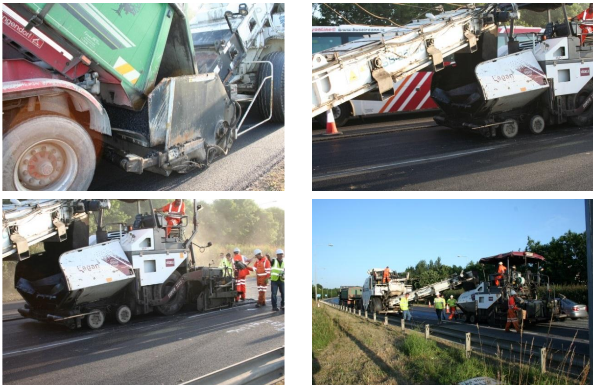
Figure 5. Paving process of the trial section
