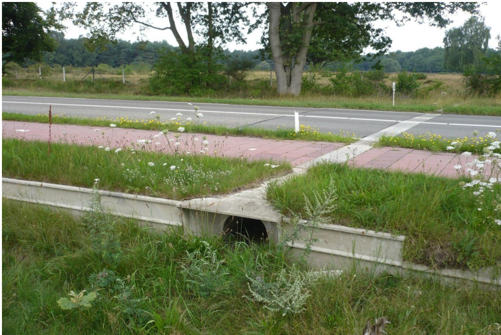
Figure 2-4 Amphibian tunnel and drift fences to help toads safely across the road. Photograph: E.A. van der Grift
