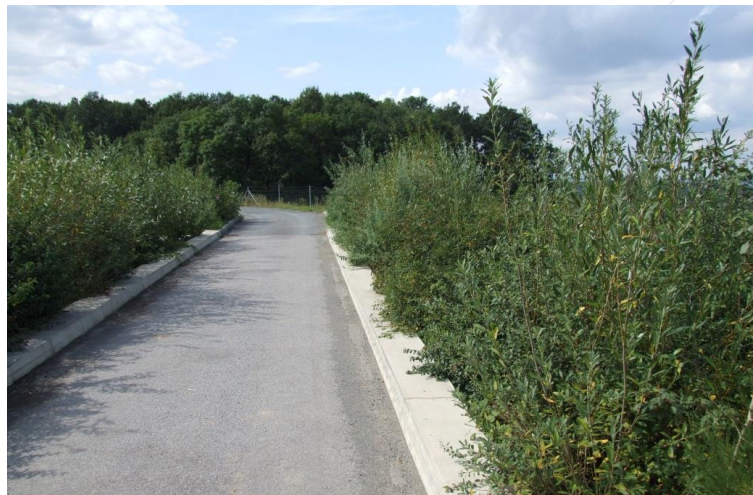
Figure 3-4 The hedgerows planted in the green verges should form an unbroken guidance structure over the bridges. Photograph by SWILD & NACHTaktiv.
