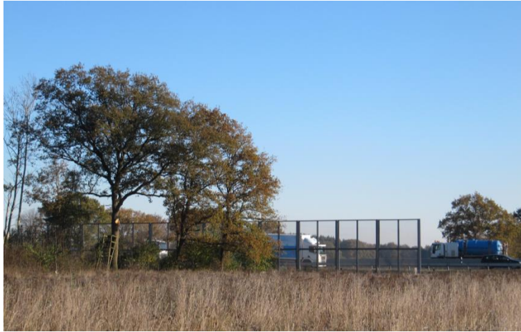
Figure 3-7 Screens or dense vegetation on road verges may encourage some bats to increase their flight height before crossing the road. However, if the distance between the screens or tall vegetation is too long, the bats may descend over the road. Photograph by M. Elmeros.
