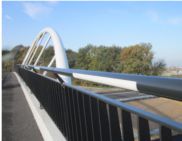
Figure 3-12 Lighting on this bicycle bridge in the Netherlands has been installed in the railing to reduce the light spillage into the surroundings and maintain a dark zone along the bridge to encourage the bats to use it as an overpass. Photograph by V. Loehr.
