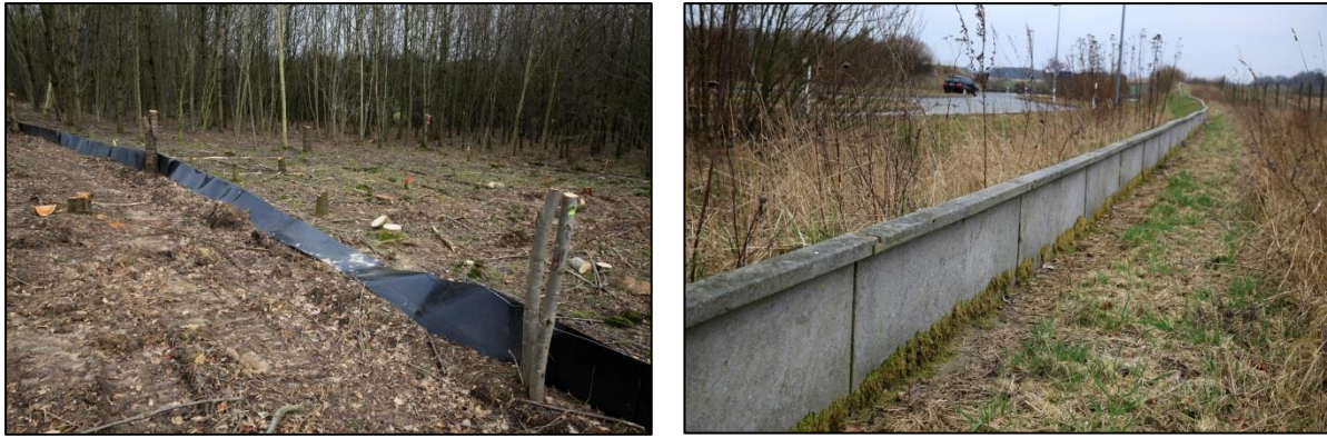
Figure 2-7 Synthetic amphibian fences (left) tend to fail a few years after installation. Concrete barriers (right) can be seen as a more robust and sustainable alternative. Photographs: E.A. van der Grift.
