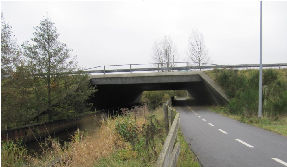
Figure 3-10 Bats may use multifunctional tunnels and culverts if there is little human traffic during the night. The underpass should preferably be unlit, and the waterway should always be maintained as a dark corridor. Photograph by M. Elmeros.
