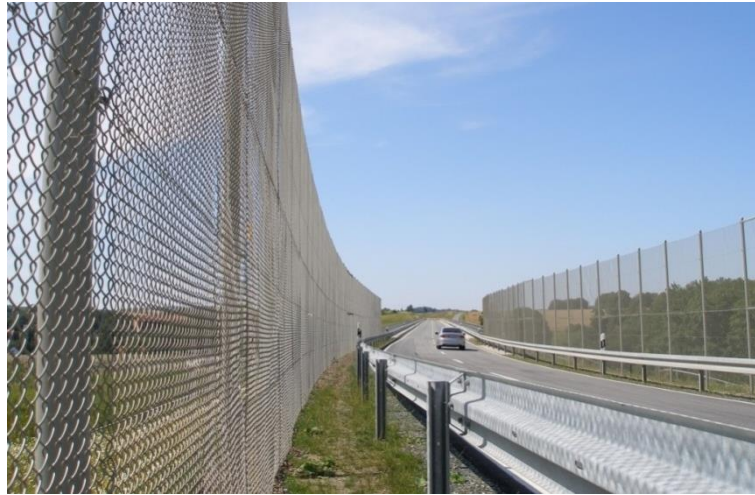
Figure 3-16 High fences are needed to discourage bat access to the road and guide them safely across road above traffic height. The illustrated fences are installed near underpasses on the state road S170n in Germany. Photograph by SWILD & NACHTaktiv.
