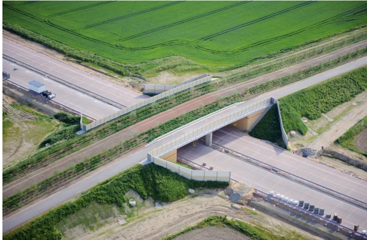
Figure 3-3 A newly constructed overbridge with an agricultural access track and planted with two hedgerows to form a flight corridor for bats across the A14 in Germany. Photograph by Landesstraßenaubehörde Sachsen-Anhalt.
