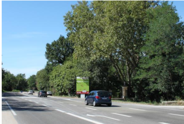
Figure 3-13 An experimental audible warning system has been installed on the regional road in France. When cars pass the patches with special asphalt (light patch under the car in the picture), a high frequency sound is generated to deter bats. Photograph by M. Elmeros.
