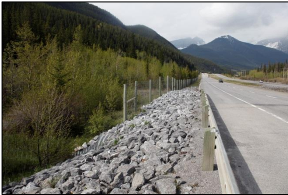
Figure 2-3 Boulder fields at the end of the fence (left) and cattle guards (right) may help prevent animals from entering the road corridor. Photographs: E.A. van der Grift.
