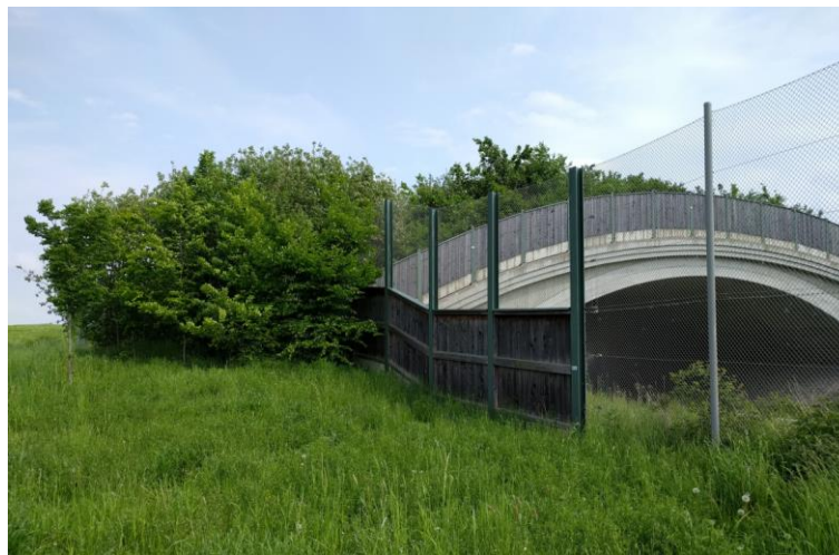
Figure 3-2 Fences and screens along the road and across the passage must be tightly connected to prevent bats from diverting on to the road. Photograph by SWILD & NACHTaktiv.
