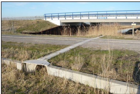
Figure 6-3 Amphibian tunnels (left) are frequently installed to help toads safely across roads during spring migration (right). Photographs: E.A. van der Griff (left) and F. Ottburg (right).
