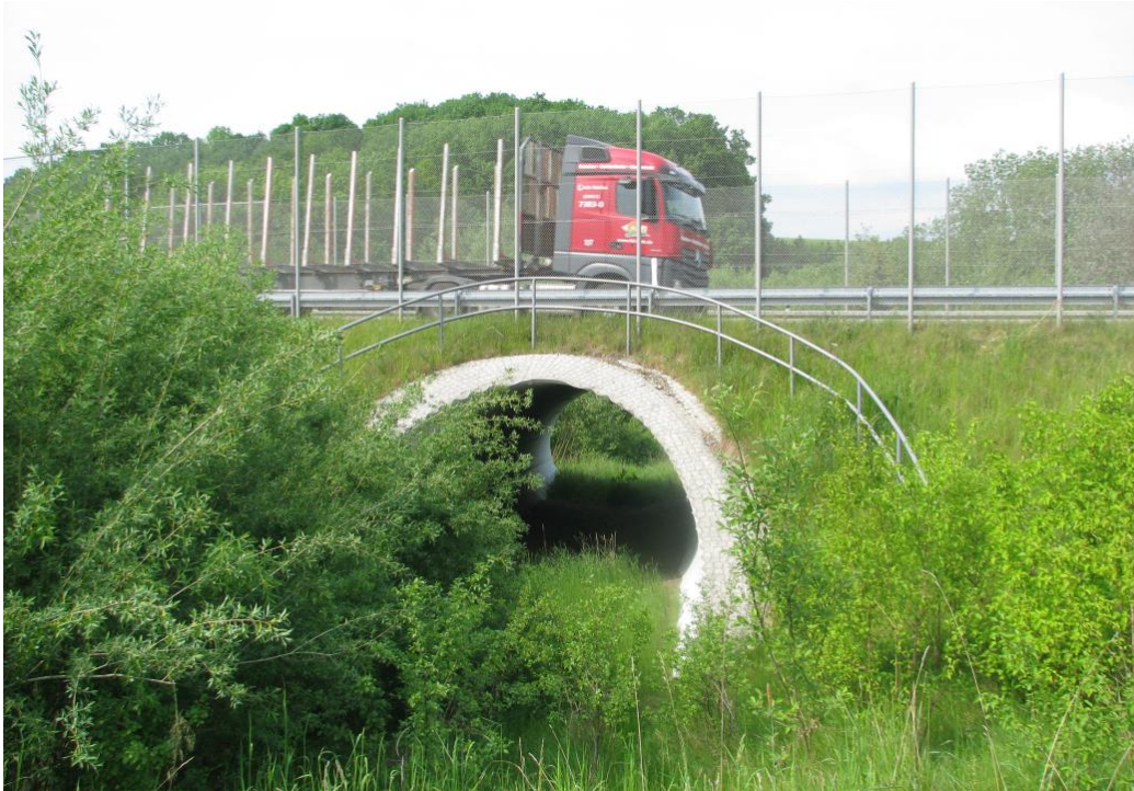
Figure 3-9 Hedgerows may guide commuting bats into the underpasses. Tall fences on the road above the underpass enhance the effectiveness of the passage for low-flying species and may function as a hop-over for species with medium and high flight behaviour. Photograph by SWILD & NACTaktiv.
