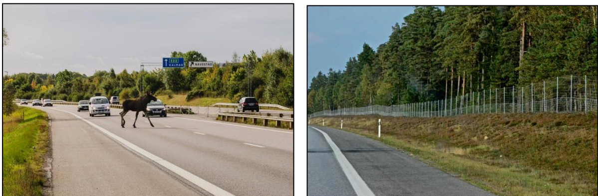
Figure 6-4 To keep moose off the road (left), wildlife fences are installed (right). Photographs: N. Luks (left) and A. Seiler (right).
