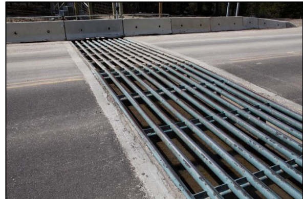
Figure 2-3 Boulder fields at the end of the fence (left) and cattle guards (right) may help prevent animals from entering the road corridor. Photographs: E.A. van der Grift.
