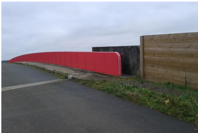
Figure 3-5 Retrofitted panels to the railings on an overbridge and a tightly fitted fence have increased the number of Rhinolophus bats using the bridge as a safe crossing structure. Photograph by L. Arthur.
