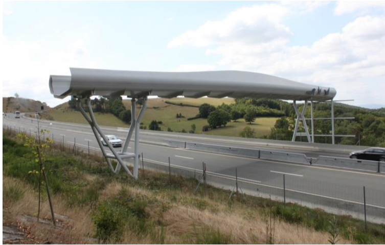
Figure 3-6 A closed-structure gantry might shield the bats slightly from traffic noise and light disturbance. The gantries must be linked to adjacent landscape elements (such as hedgerows) used by bats as a flight route. Adjacent to the newly constructed gantry shown, the vegetation has not yet developed. Photograph by M. Elmeros.
