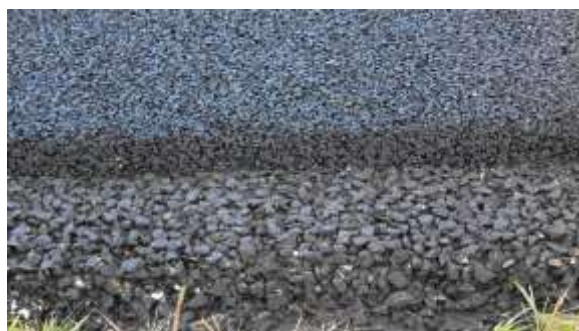
Figure 1: Example of two-layer porous asphalt
