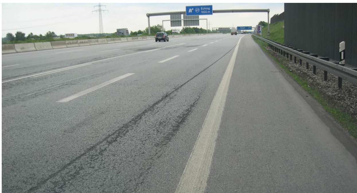
Figure 5.9: Older porous asphalt with significant ravelling in Bavaria, Germany.
