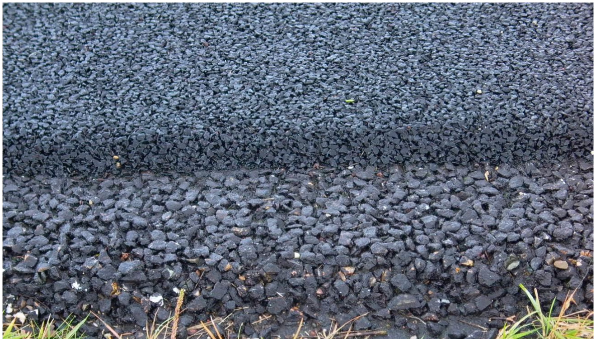
Figure 5.8: Two layer porous asphalt on a Dutch motorway seen from the roadside. The top layer has a smaller aggregates size of 6 or 8 mm, the bottom layer has 16 mm aggregates.
