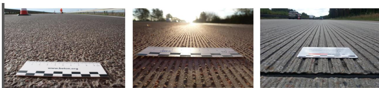
Figure 5.12: Examples of different surface treatments of concrete roads. To the right, longitudinal grinding.
