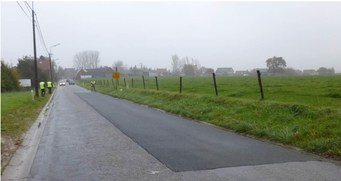
Figure 5.15: A 40 m long and two month old test section with poroelastic pavement in one lane at Herzele in Belgium [14, 27].
