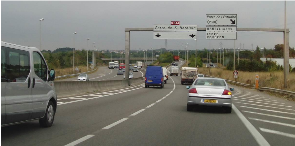
Figure 4.15: Motorway with a noise-reducing thin layer pavement around Nantes in France.
