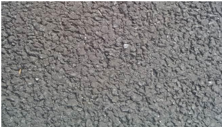
Figure 5.6: Close-up picture of the Austrian SMA-LA pavement used for noise reduction.
