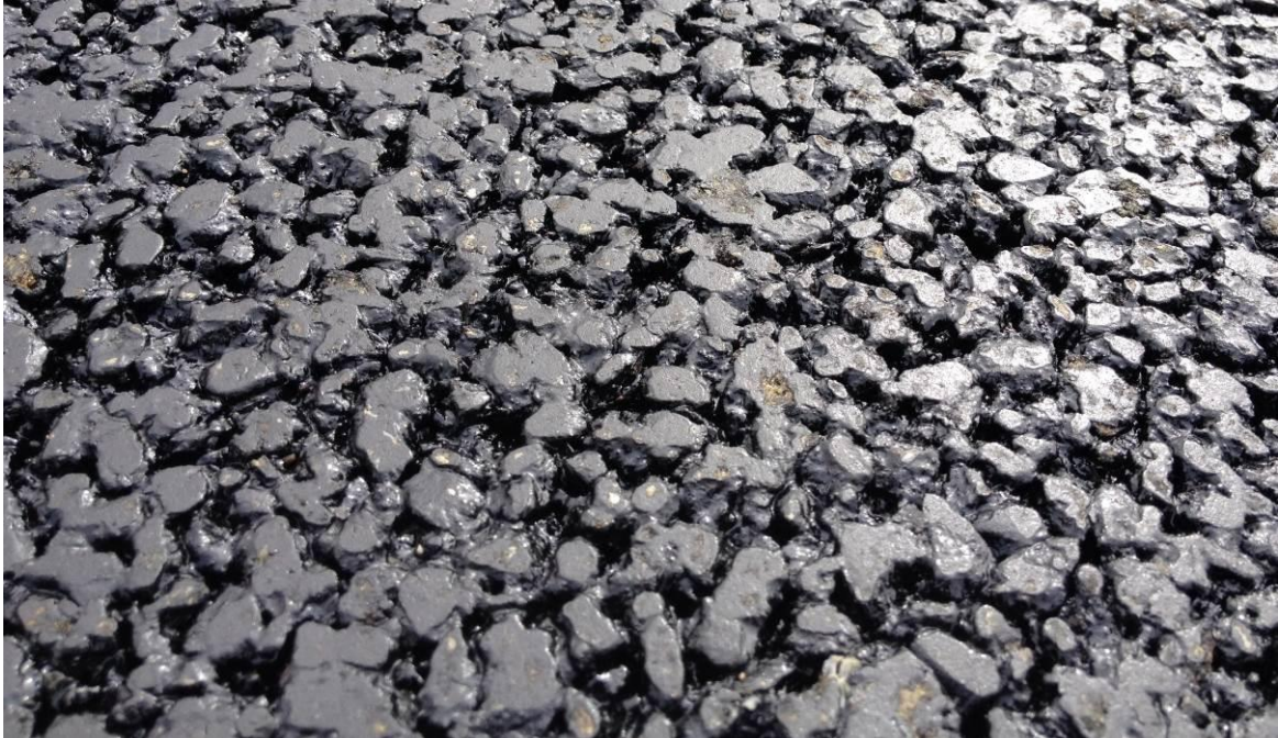
Figure 4.6: Close-up photo of a newly laid SMA pavement with a very smooth and even surface texture that reduces vibration generated noise. Open cavities in the pavement surface can also be observed. These are helping to reduce the noise generated from air pumping.
