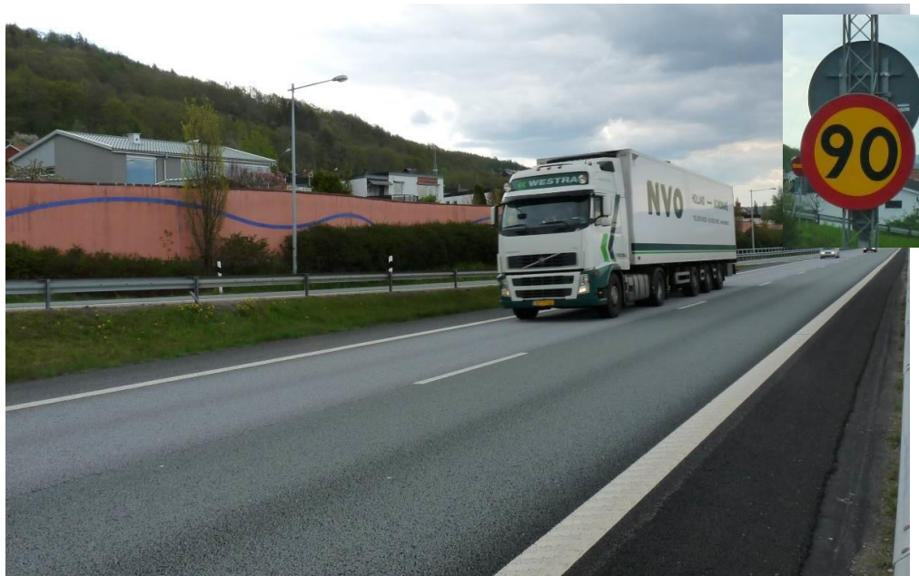
Figure 5.11: At motorway E4 in Husqvarna in Sweden a combination of noise-reducing pavement, noise barriers and speed reductions have been applied to fulfil noise guidelines.
