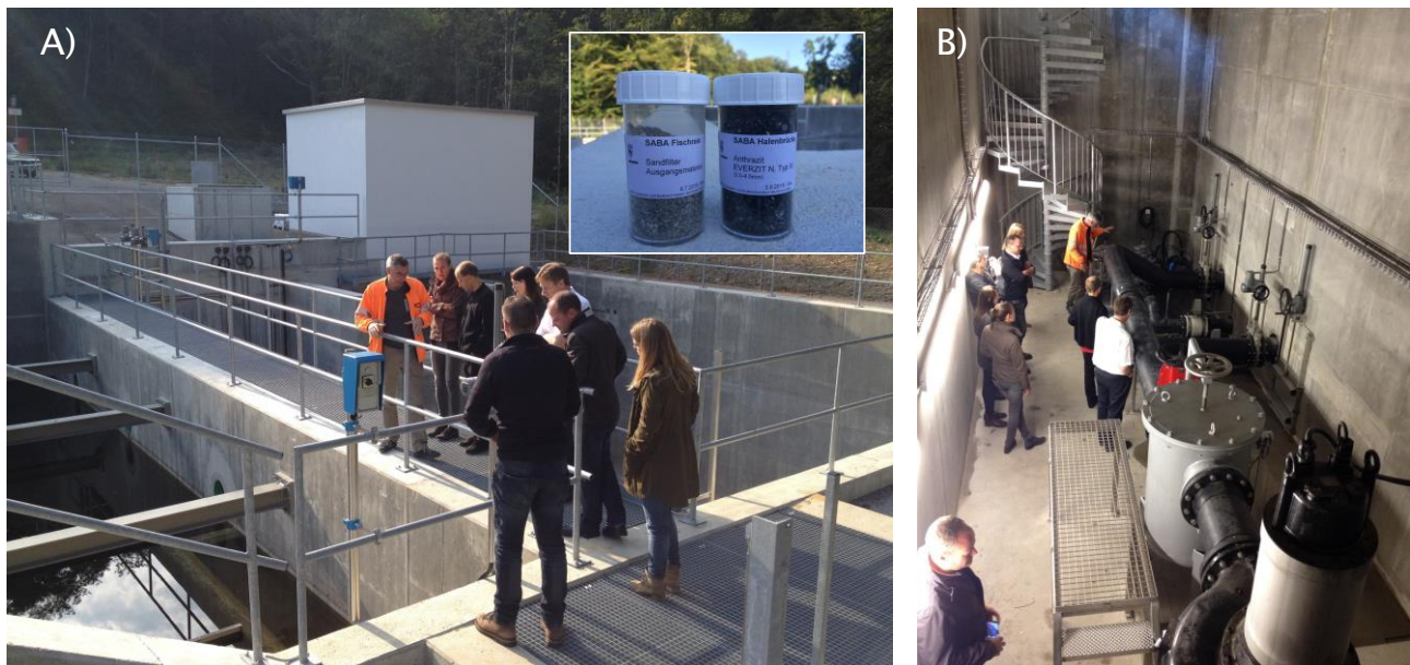
Figure 15: The advanced technical treatment system at Halenbrücke, Switzerland. The plant was opened in 2015 and receives runoff from 18 km of roads with an ADT of approx. 90,000 vehicles/day. The treatment is based on storing, sedimentation, and one-step filtration with active carbon (anthracite). The capacity is 60 l/second. The system cost €4.8 million to build. A) At the basins. The insert shows filter material (the sand material on the left is used in another newly built treatment plant). B) Inside the treatment plant (photo: Sondre Meland)
