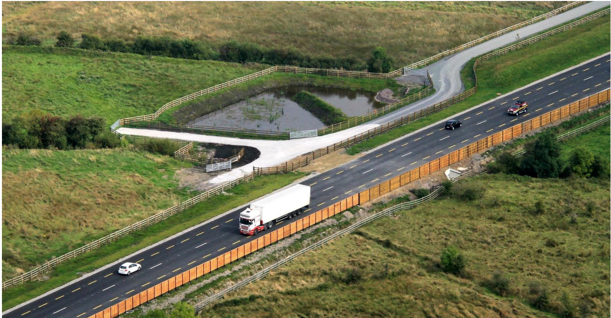
Figure 12: Example of SUDS in Ireland. Combined wetland, sedimentation, and attenuation facilities (photo: Transport Infrastructure Ireland)
