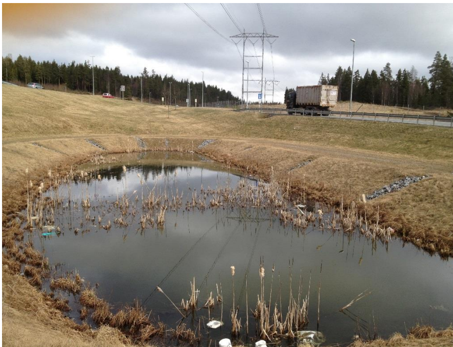
Figure 17: Example of a Norwegian sedimentation pond with a smaller pre-sedimentation pond (forebay, which can be seen in front of the band of vegetation crossing the pond) and a main pond (photo: Sondre Meland)
